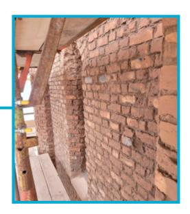
Photos showing an airtight encapsulated work area at Coolderry railway bridge, both during and post grit blast cleaning.
