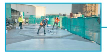
Photo shows application of chemical protective coating Brenntag, Belfast.
